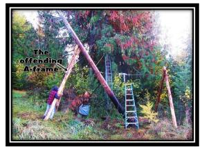
this operation using one man, 3 females, and 1 boy to lift a pole (so heavy that it took several of us to roll it -- it was about 16 in. in diameter at the bottom) to a 90 degree angle, into the upright position to slide it in the pre-dug (by hand)
